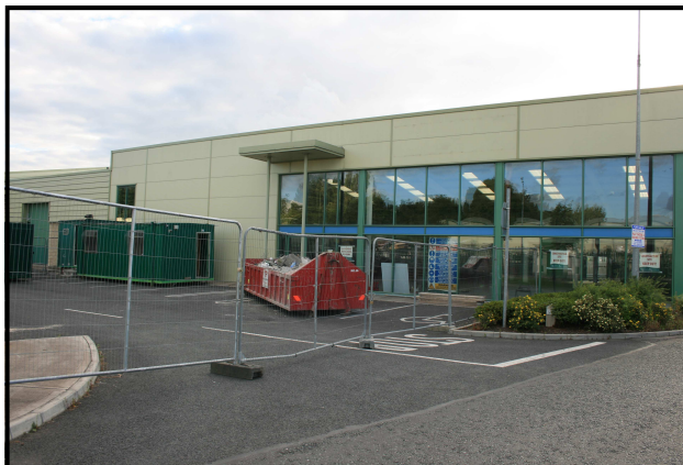
Building Work has commenced at the school.
